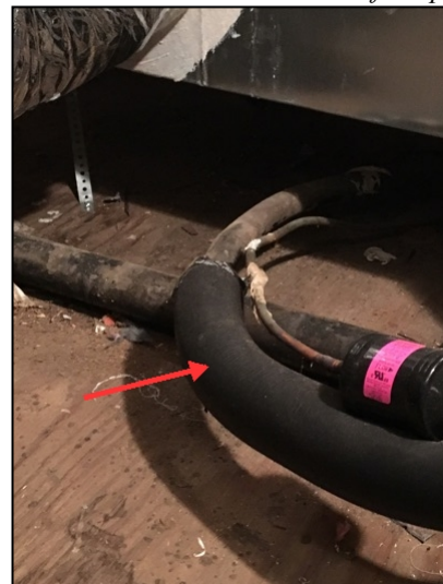
Recommend replacing the old refrigerant line insulation with newer insulation as already installed on a section of refrigerant line near the AC unit in the attic
