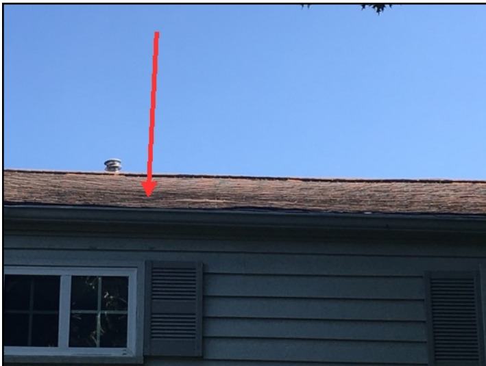
Roof deflection on the front side of the roof
