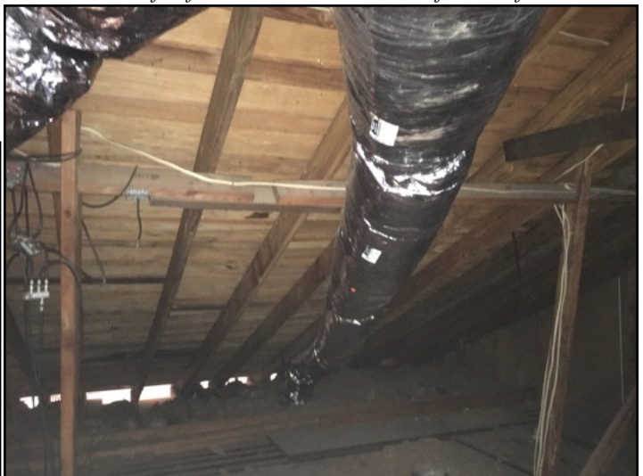
Inadequate purlin bracing
