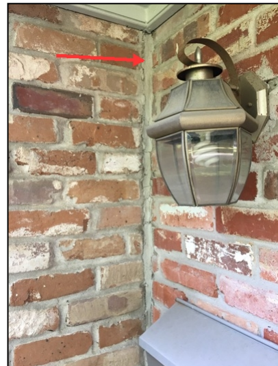
Mortar patch at the front left corner
