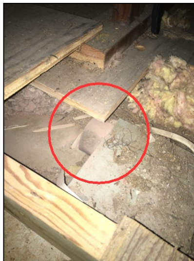
Both upstairs bathroom exhaust fans were improperly venting to the attic, which allows moist air into the attic
