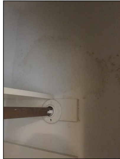
Observed stains/corrosion on the interior walls of the upstairs hallway closet
