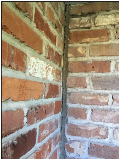
Mortar patch at the front right corner
