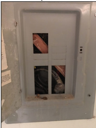
Sub panel behind the refrigerator had open knockouts and exposed cables. This appeared to be a discontinued panel
