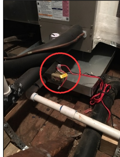
Float switch installed on the overflow pan
