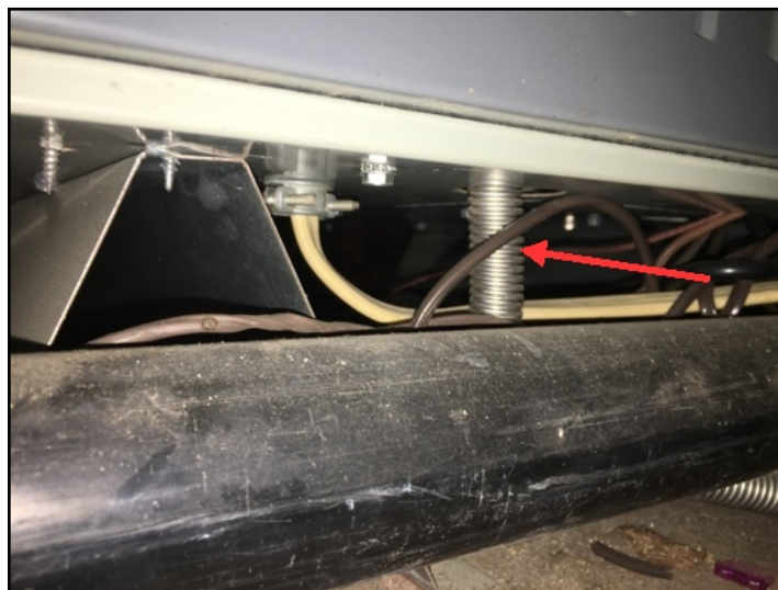
The flexible gas connection for the furnace passed through the enclosure cabinet
