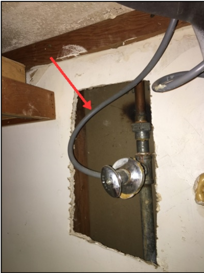
Observed improper material (appeared to be rubber) used for the flexible water line connections in the upstairs bathroom lavatory
