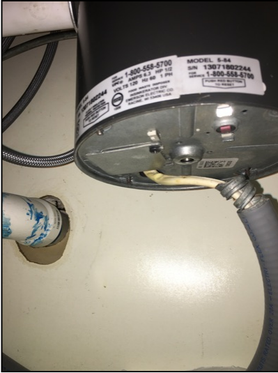
The waste disposer had no electrical stress connector/strain relief clamp
