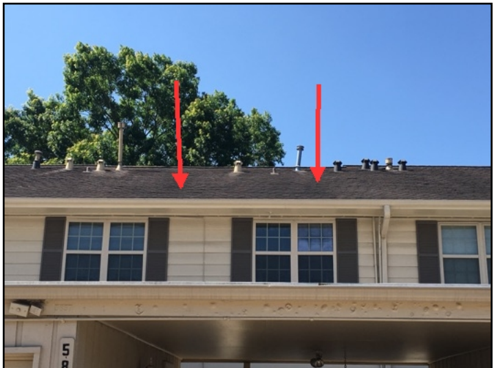
Roof deflection on the back side of the roof
