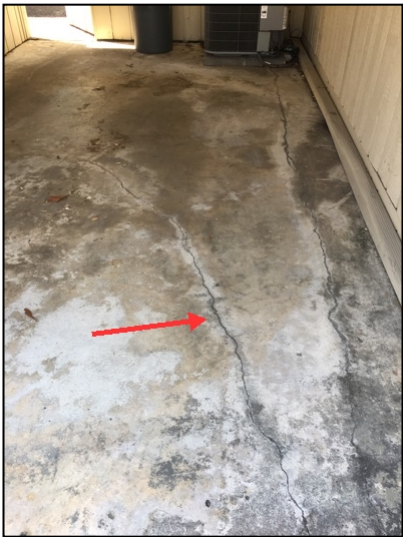
Cracks in the carport slab
