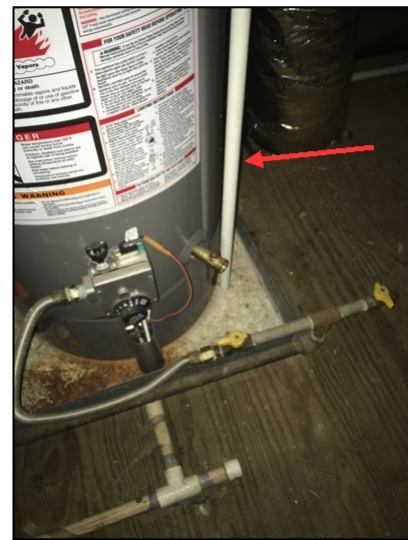
Water heater TPR valve discharge line
