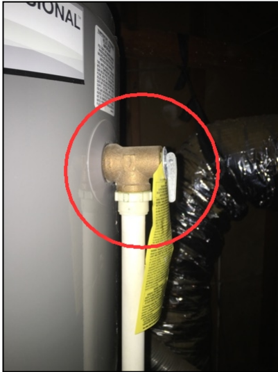
Water heater TPR safety valve
