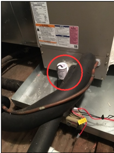
Float switch installed on the overflow outlet at the primary pan
