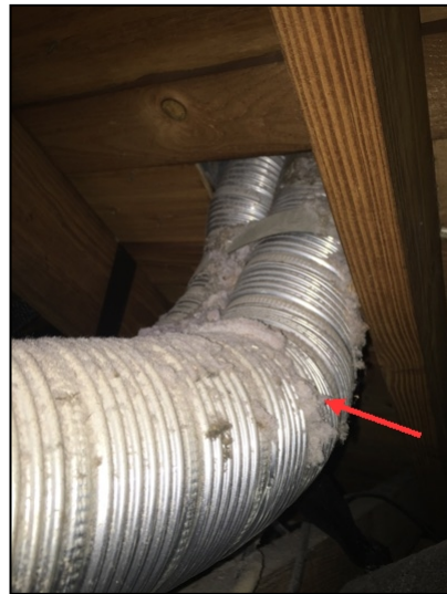
The dryer vent was venting lint in the attic
