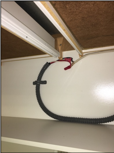
Exposed splice wire for the cooktop
