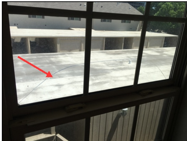
The upstairs back left bedroom window was cracked
