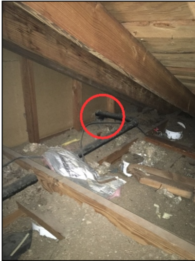
Penetration of the firewall between townhomes
