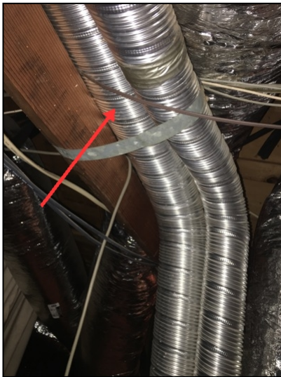
Dryer vent should be hard walled
