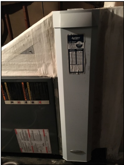
Media air filter in the attic
