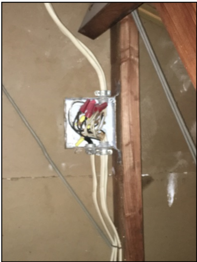
Exposed junction box in the attic
