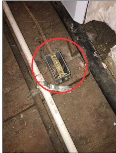
Exposed junction box (furnace switch) for the furnace wiring
