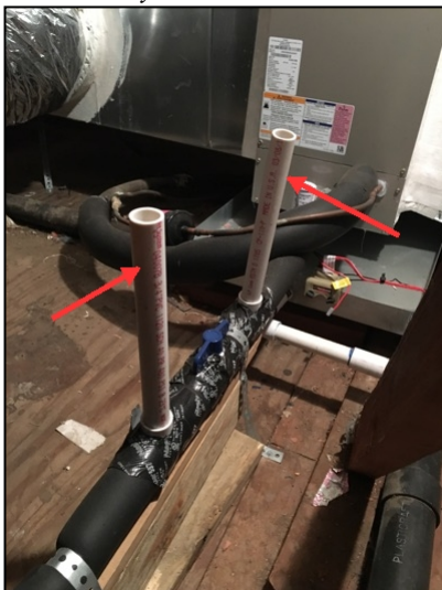
Primary condensate drain line clean outs in the attic
