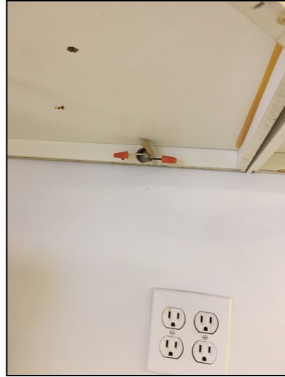
Exposed splice underneath the kitchen cabinet
