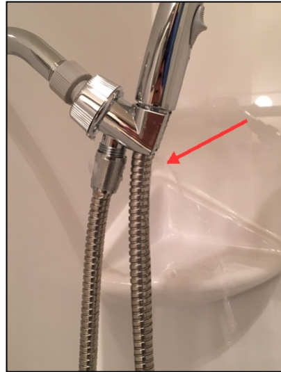
The shower head in the upstairs bathroom was leaking.
